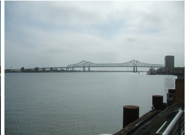
Bridge over Mississippi River.
