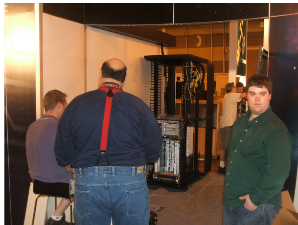
In background is the mostly empty network-demo rack.
