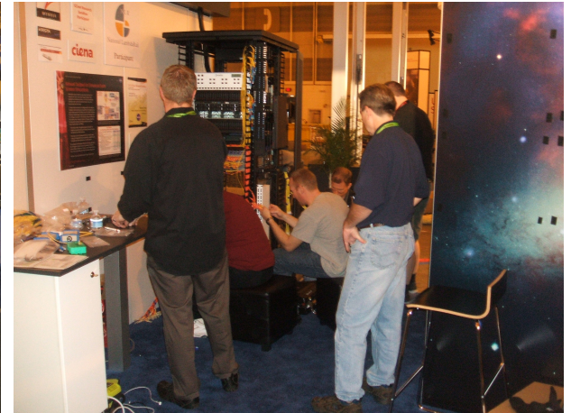
Lots of network equipment to to unrack in the NASA Exhibit Booth.
